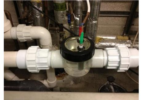
Using a pair of pliers, carefully unscrew the electrodes from the lid. Always ensure when replacing the electrodes, the rubber seal is placed against the lid followed by the plastic washer then the electrode nut. Please contact your supplier if any of these parts need replacing. When replacing the lid, make sure the lugs are in line before pushing the lid onto the chamber.
