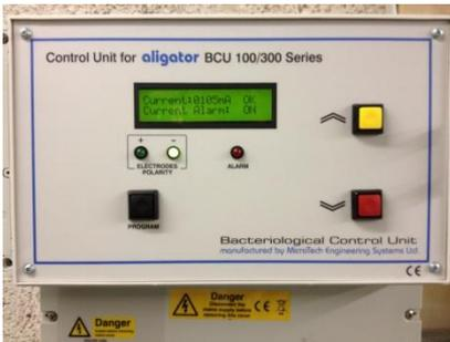
Mount the BCU on the wall as close to the electrode chambers as is practical. The outside case of the unit is IP65 (IEC 60529:1989) rated, so is therefore splash proof. The display on the controller is sensitive to viewing direction. It is designed to be read from a  $45^{\circ}$  above the horizontal and  $10^{\circ}$  below the horizontal. Therefore mounting the controller to high or low will result in the data on the display being unreadable.
